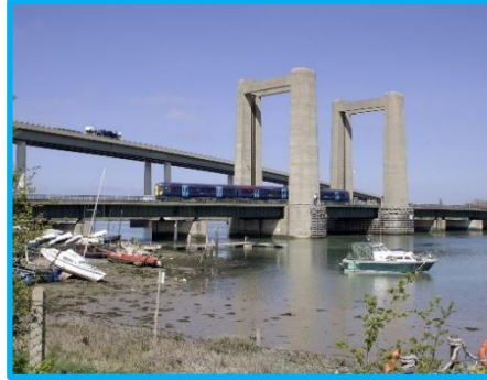
Class 375 on Kingsferry Bridge Courtesy of Dominic Noades
