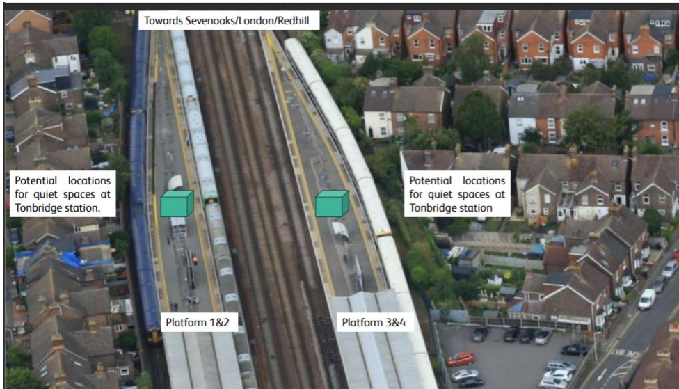
Figure 37 Potential location of quiet spaces at Tonbridge station. Source: Network Rail.
